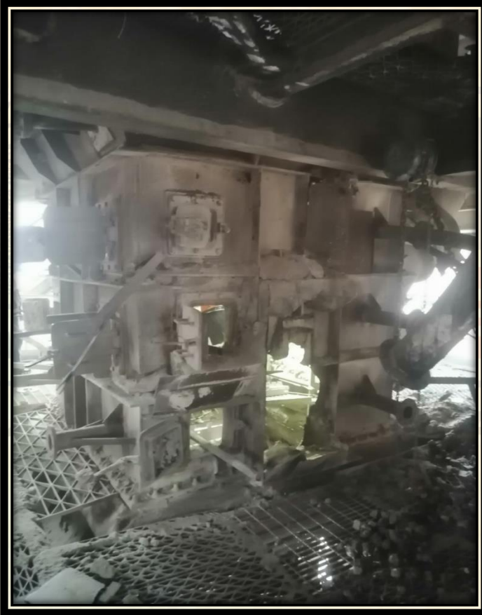
Dismantling of Existing smoke chamber
